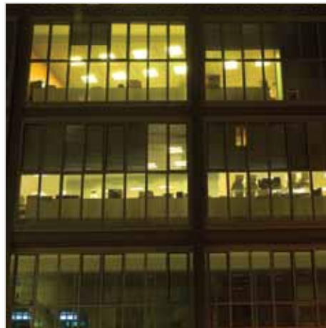
Achievement of a four-star Green Star South African rating for energy efficiency
