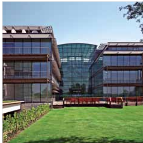
17 integrated sequences, which improve building efficiency
