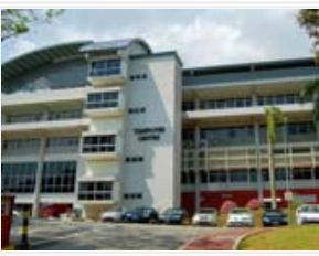
Computer Centre Primary Data Centre
