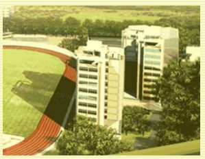
NUS High School Secondary Data Centre
