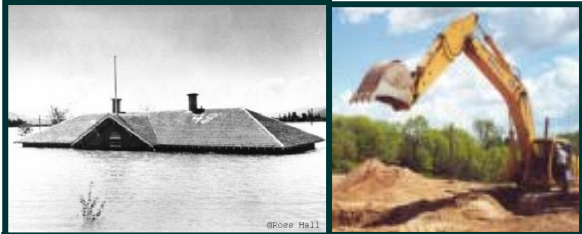
Loss of Headquarters or Campus
